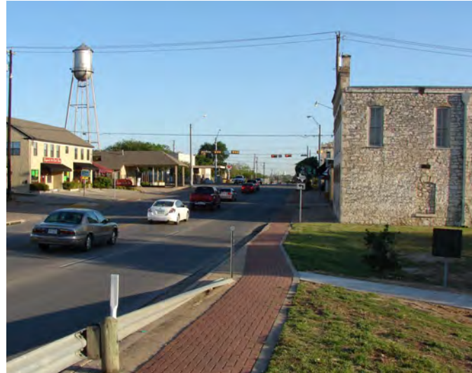
South Mays Gateway: Existing
