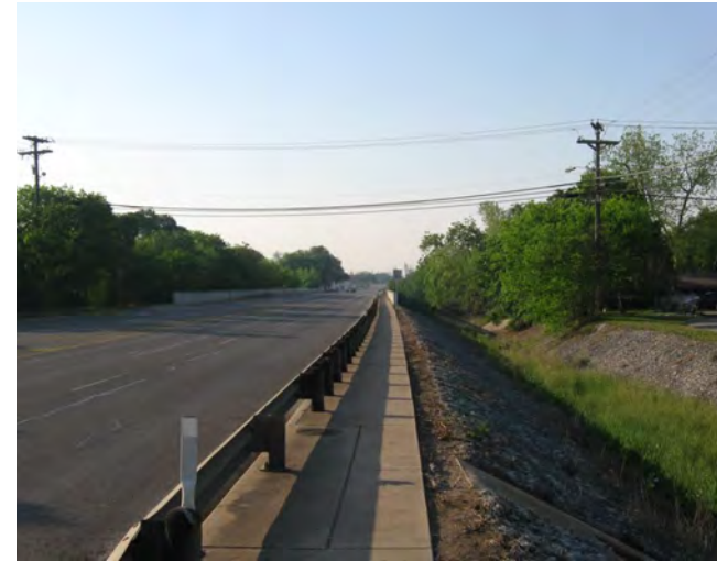
North Mays Gateway: Existing
